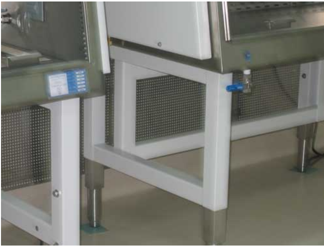
HEPA filters in biocontainment facilities are often incorrectly mounted beneath biological safety cabinets. In this instance, air cannot reach the filter in a proper manner. (Photo courtesy of Tony Della-Porta.)
